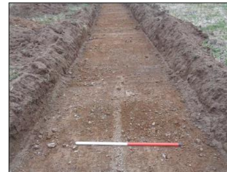
Plate 67. Trench 17, geophysical anomaly (gravel and stone), from NE
