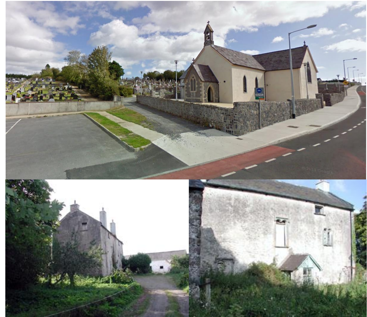
Figure 10.2 Saint Mary's Catholic Church and Ballygunner castle, Knockboy, County Waterford (Source: Google 2019, http://www.buildingsofireland.ie )
