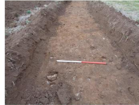
Plate 11. Trench 3, patches of stone and gravel (geophysical anomalies), from ESE.
